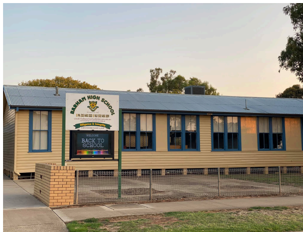
Front of BHS
